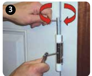
When in position secure the socket screw. Take care not to overtighten. Replace the covers.
