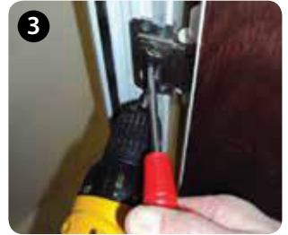
Secure the screws in the side plate.
