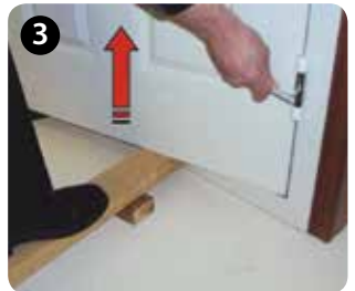
Lift and support the door to the required height whilst securing the socket screws. Take care not to overtighten. Replace the covers.
