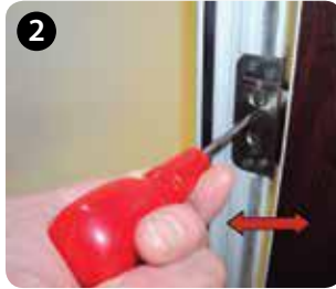
Lever the slide plate (B) with a screwdriver in the adjustment slot
