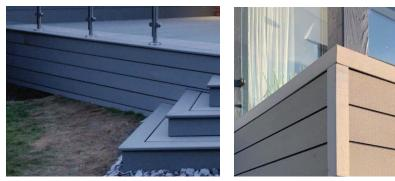
Cladco Composite Fascia Boards can be installed using both Sumo Grip Adhesive and 50mm Speeddekz Screws. When installing alternate between Sumo Grip and Screws every 150mm until the Board is firmly in place. The supporting structure underneath the decking must have adequate supports for the fascia board to be secured into. Sumogrip alone will not support the weight of the board and must be used in conjunction with screws.
