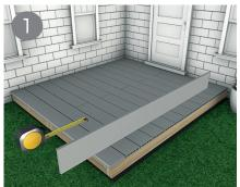
Measure the edge of the decking area to obtain the length required, skirting trim can be cut to size as needed. If you need a longer length than 2.2m simply butt the two skirting edges up together.
